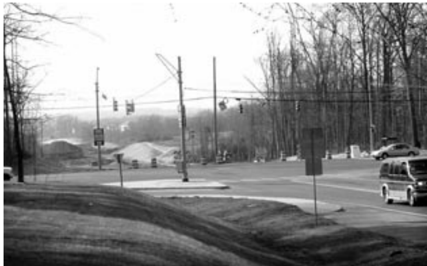
Extensive clearing for the 28/198 extension at New Hampshire Avenue.
